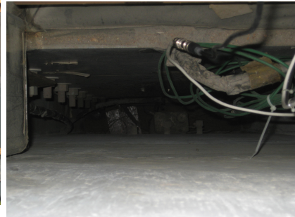
Figure 4: Vertical shaft found in room 275, where the large liquid scintillation tank sits. See larger image here
