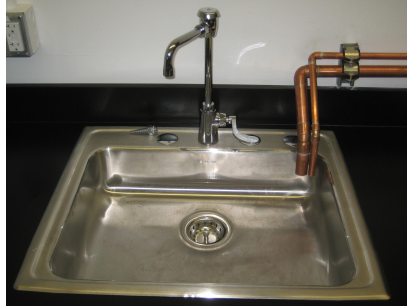
Figure 8: Water drains Click here to see larger picture
